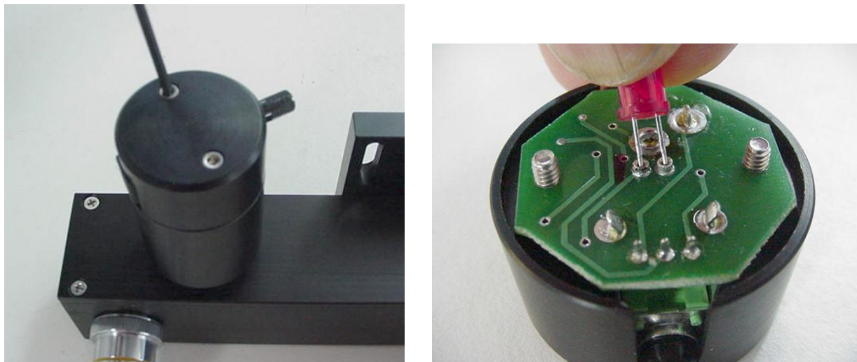
Figure 5: a) Removing the LED lamp housing; b) replacing the LED.
